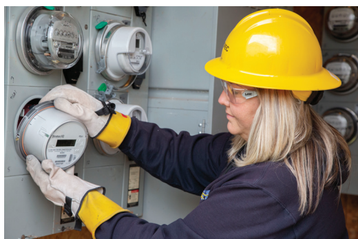
NOVEC Field Services Technician Candace Burns installs an advanced meter at an apartment building in Manassas.
