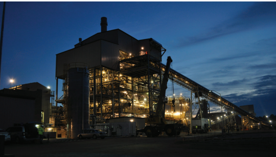
The Biomass Facility, which celebrated its 10th anniversary in 2023, is managed by NOVEC Energy Production, a NOVEC subsidiary. The plant produces 49.9-megawatts of renewable energy, enough to power 16,000 NOVEC homes.
