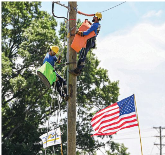
Journeyman Blake Sparling and Zack Bell perform tasks on the pole while teammate Brian Savage (not pictured) monitor work from the ground. Photo by Jim Robertson.
