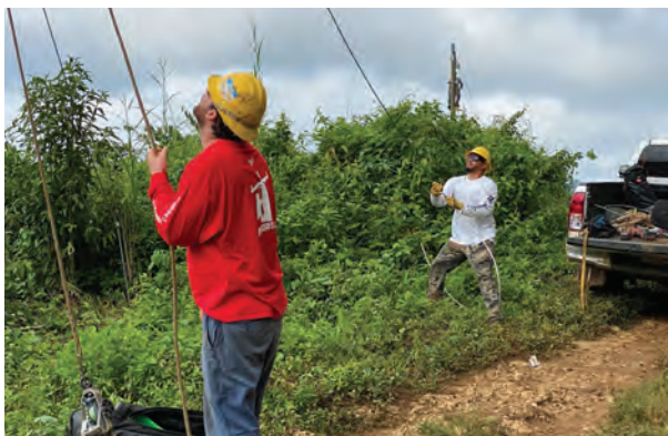
Lineworkers Blake Sparling and Mauricio Paz (right) work to bring electricity to the residents of Santa Isabel, Guatemala.
