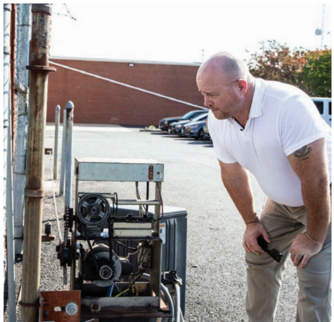
Luke Cassidy checks on the operation of the security gate at one of NOVEC's Manassas locations.
