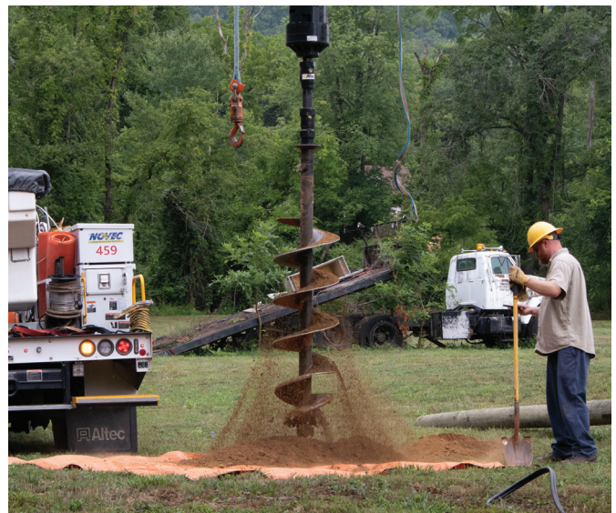
NOVEC prepares to install a new electric pole in Loudoun County.
