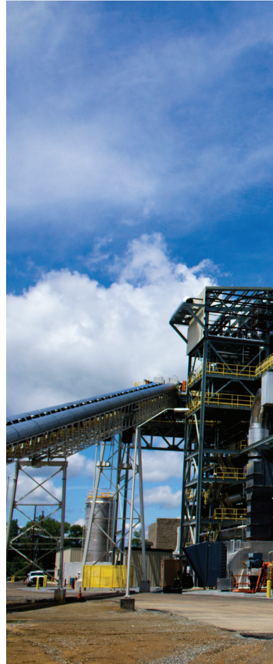
NOVEC's Biomass Facility located in Halifax County. Photo by NOVI Energy.
