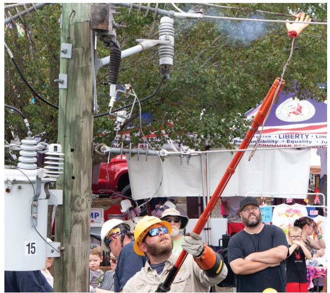
Casey Taylor, NOVEC line technician 2nd class, shows the gathering crowd what happens when a glove touches an energized wire — it catches on fire.
